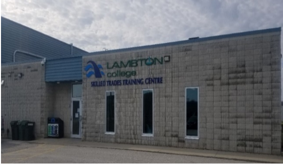
Picture 10. Skilled Trades Training Centre (STTC)
