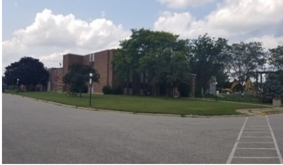
Picture 8. North Building
